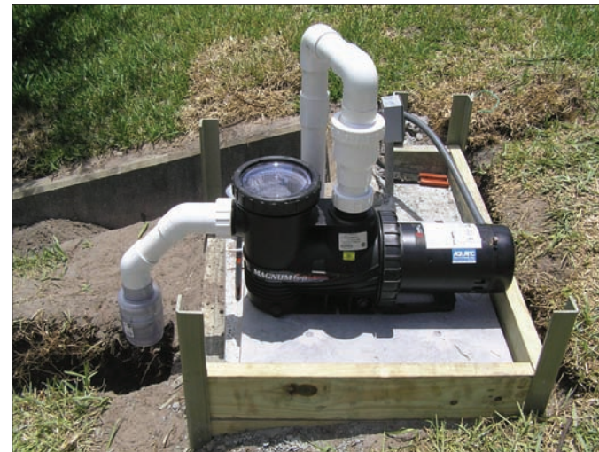
Example of Onshore concrete pad.
